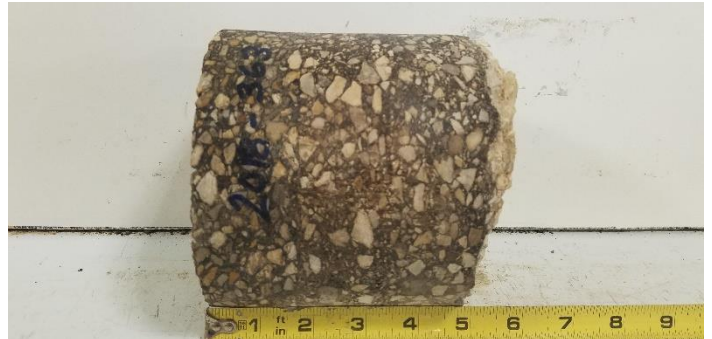
Asphalt Core from Boring B-8 North of S. PanAm Expy Over Broadway St At Southbound Right Lane
