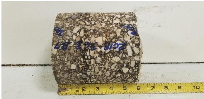
Asphalt Core from Boring B-7 North of Broadway St and Pearl Pkwy Intersection At Northbound Left Lane
